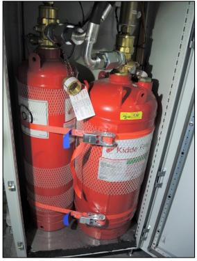
Figure 26: Novec cylinders in the port technical room. The smallest cylinder on the left is for the battery room while the cylinder on the right is for the engine room. Gas from both cylinders was released. Photo: NSIA
