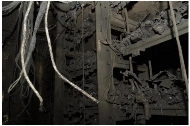
Figure 31: Damage to the battery room, seen from the battery room door. From left to right: battery stacks 3 and 2. Battery stack 1 (next to battery stack 2) cannot be seen in the photo. Photo: Kripos
