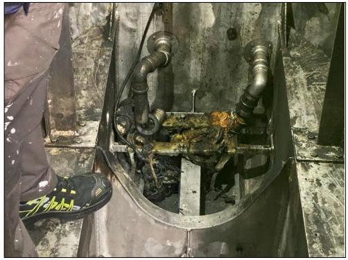
Figure 8: The greywater tank was located under the sole of the battery room. Photo: The insurance company
