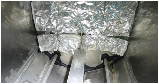
Figure 23: Fire insulation almost all the way to the bottom of the vessel, with SIKA Firestop at the lower end. Photo: NSIA
