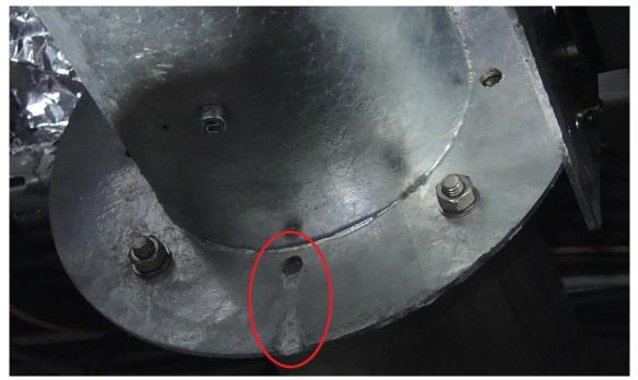
Figure 42: Salt deposit at the bottom of the flange for the fire damper in the ventilation outlet. Photo: NSIA
