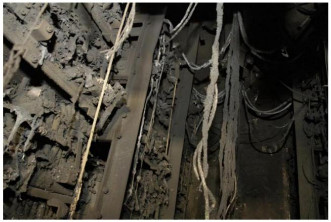
Figure 30: Damage to the battery room, seen from the battery room door. From left to right: battery stacks 6, 5 and 4. Photo: Kripos
