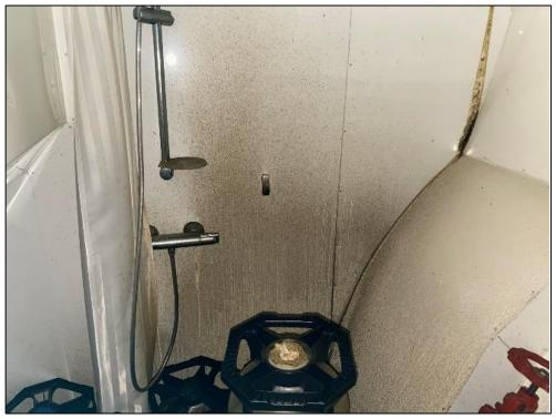
Figure 7: Clear traces of high temperatures having damaged the wall adjacent to the battery room. Photo: The insurance company
