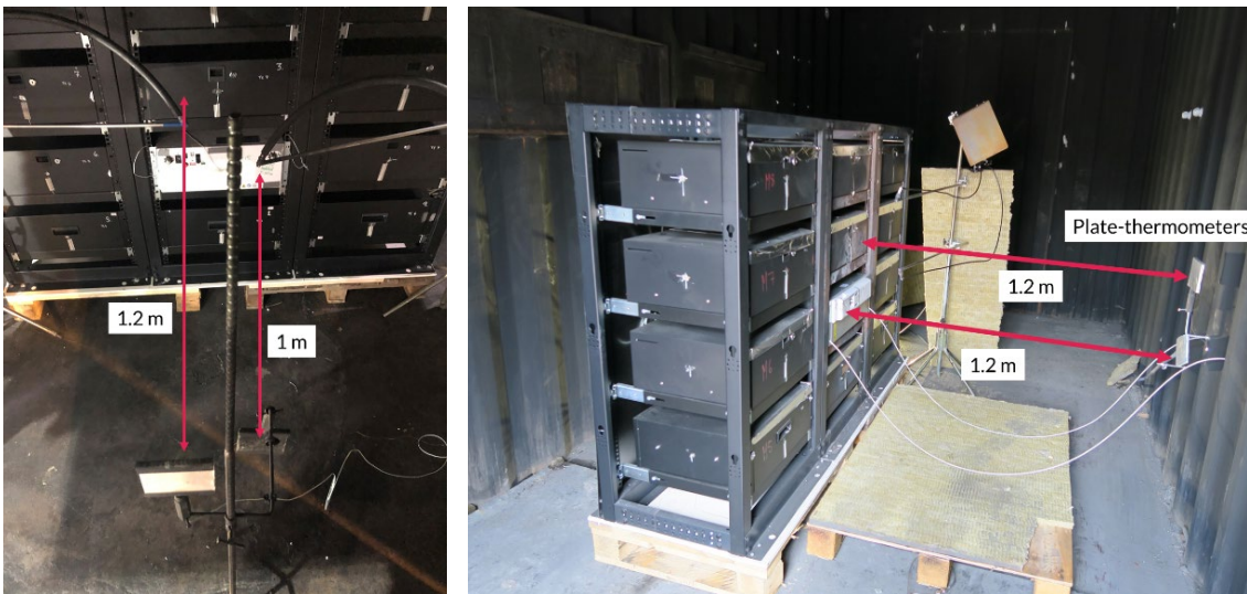
Figure 16 Location of plate-thermometers, indoors (left); outdoors – shipping container (right)
